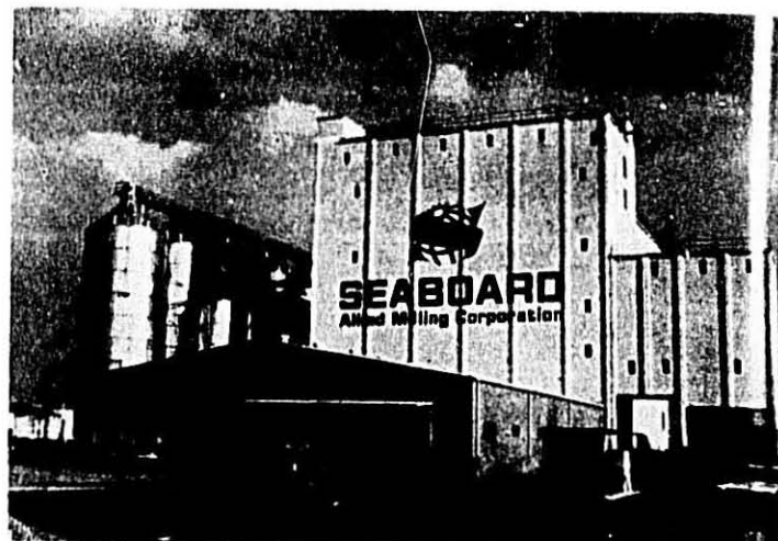
Seaboard Allied Milling Corporation's new mill at Albany, New York as it nears completion.
