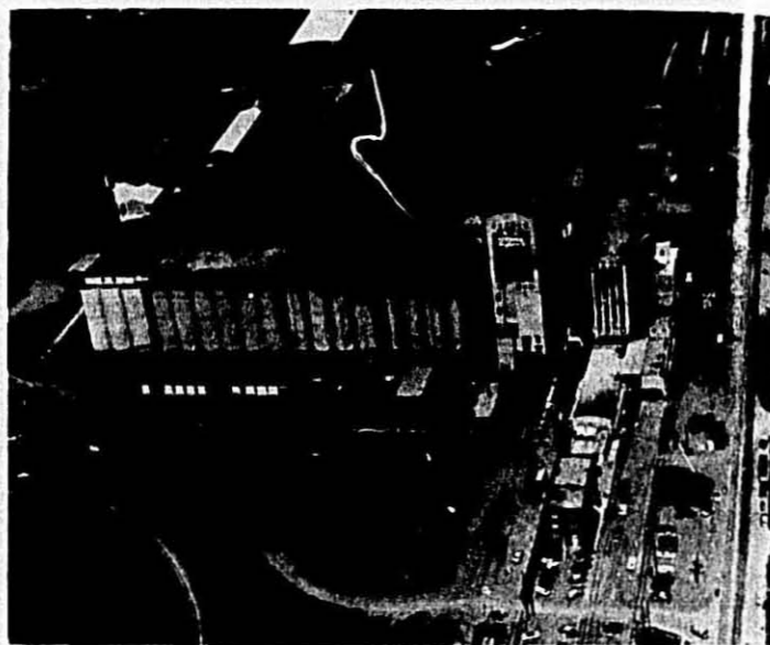
North Dakota Mill & Elevator, Grand Forks.
